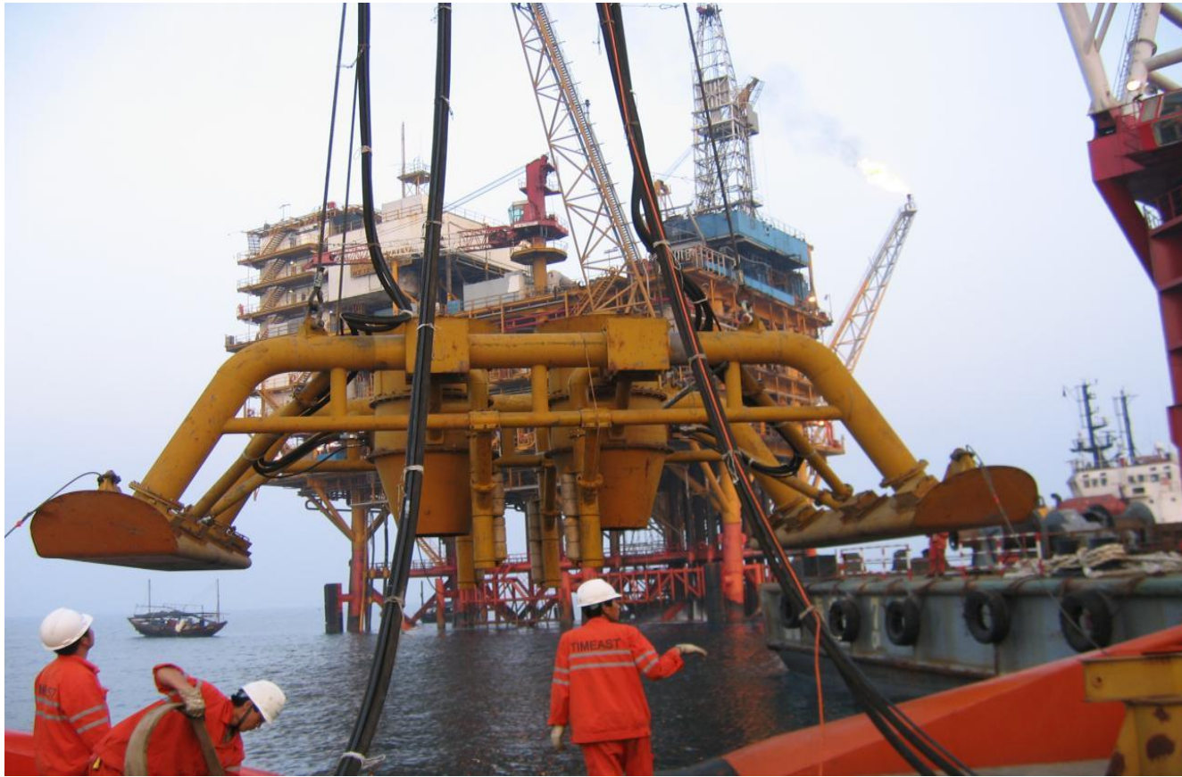
Operation On Site
